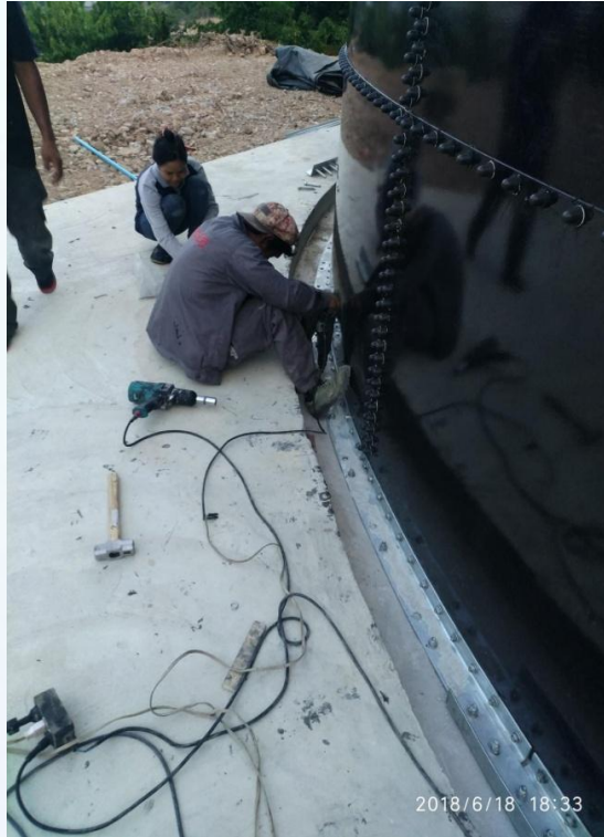
Install the base angles
