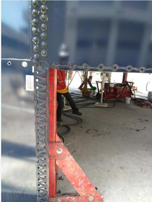
Apply the Sealant
