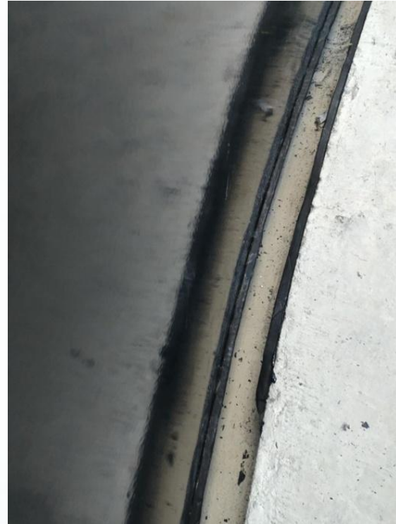
Water-expanding rubber strip
